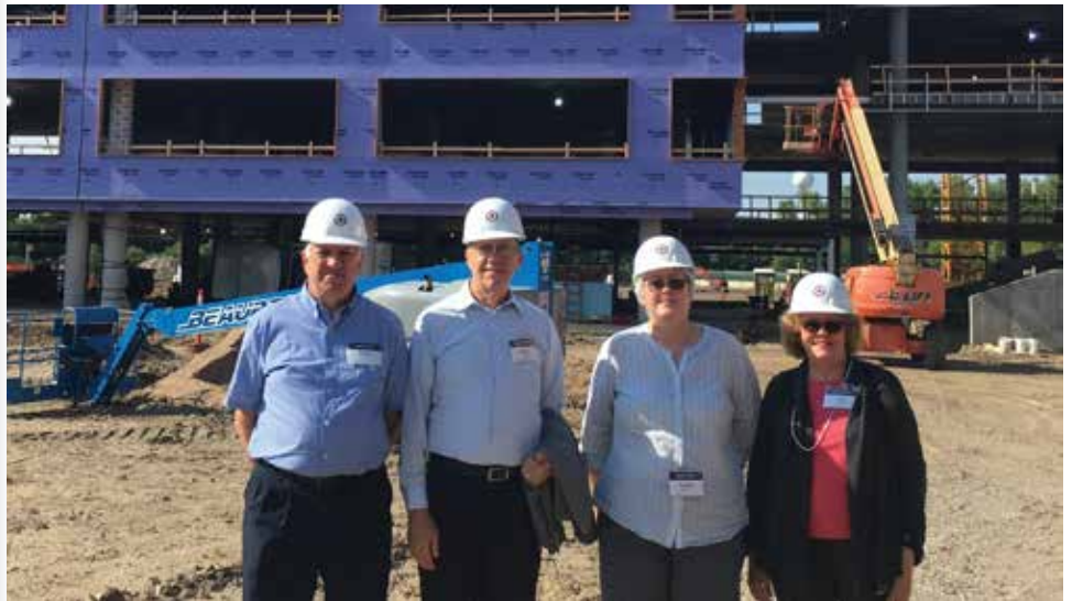
Mayor David Grant and City Council members Steve Scott, Brenda Holden and Fran Holmes toured the construction at the Land O' Lakes expansion site in July along with Land O' Lakes executives and team members from McGough construction.
