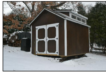
SHED AT 4073 VALENTINE COURT CITY OF ARDEN HILLS, RAMSEY COUNTY, MINNESOTA.
